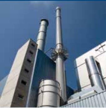
**Cogeneration of heat and energy** Since both electricity and heated steam are required for paper manufacturing, papermills running in-house thermal power stations rely on the cogeneration principle – one of the most efficient concepts available for utilising primary energy. This option is being adopted by 72 % of all papermills in Germany, making the paper industry the only sector where this practice is implemented so consistently.
